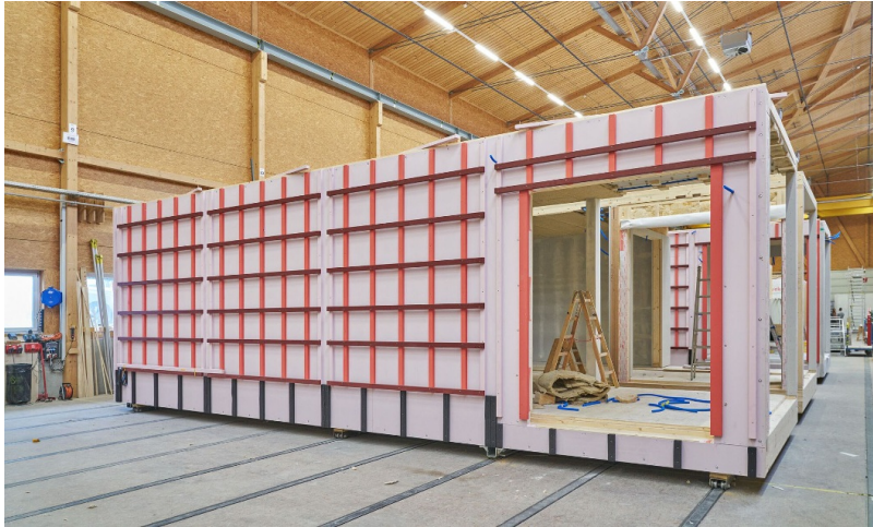
Production of modules for school building Hohlstrasse
