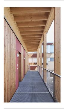
The school building is accessed via an arcade, which saves on building mass and provides adequate fire protection.
