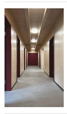
The walls and the monopitch roof were realised in timber frame construction.
