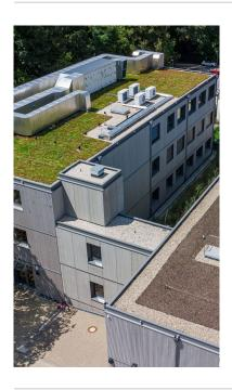
The bottom two floors were built at the German plant in Grossenlüder and the top floor the top floor at Erlenhof in Switzerland.
