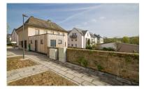
The new building with public toilet and utility room consists of just one timber module and fits perfectly between the existing building and the wall.
