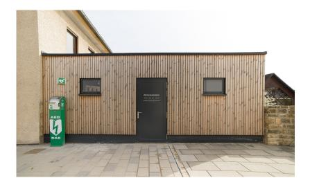
Harmonious addition: with its facade made of untreated, planed TMT, the modular timber construction also blends in well with the colours of its surroundings.
