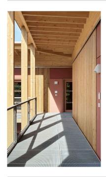
The two structures of the modular timber construction are accessed and connected by arcades.
