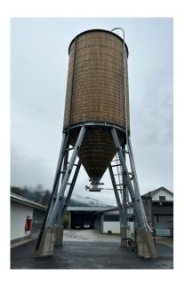
Silo outlet with double segment gate valve, emergency inspection gate valve and height-adjustable windsock
