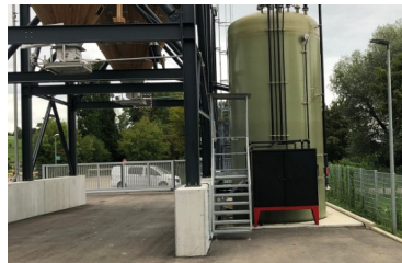
Side view of the silo facility in Uhingen
