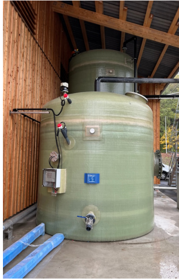
Salt silo made of larch wood with brine system
