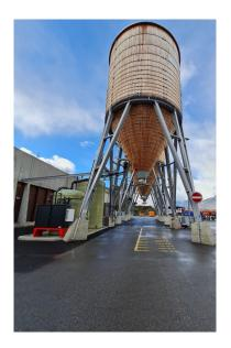
Silos with 400 cubic volume with brine generator
