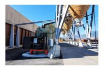
Salt exhaust with screw and rinsing cyclone
