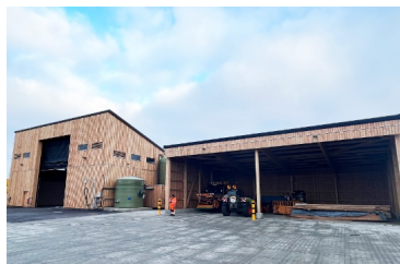
Brine facility on Sylt
